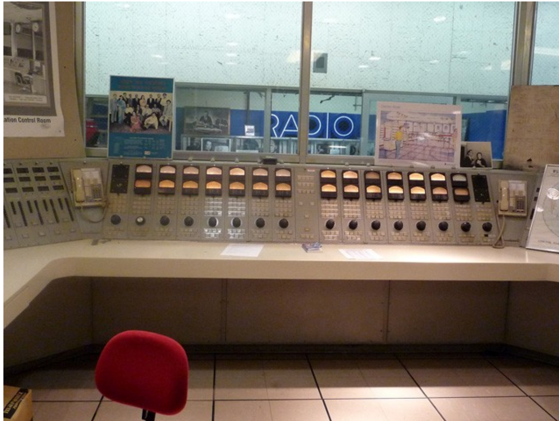
Meters & faders for program feeds to multiple regions
