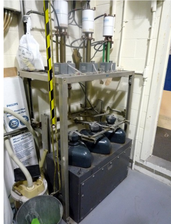
Voltage/current transformers
