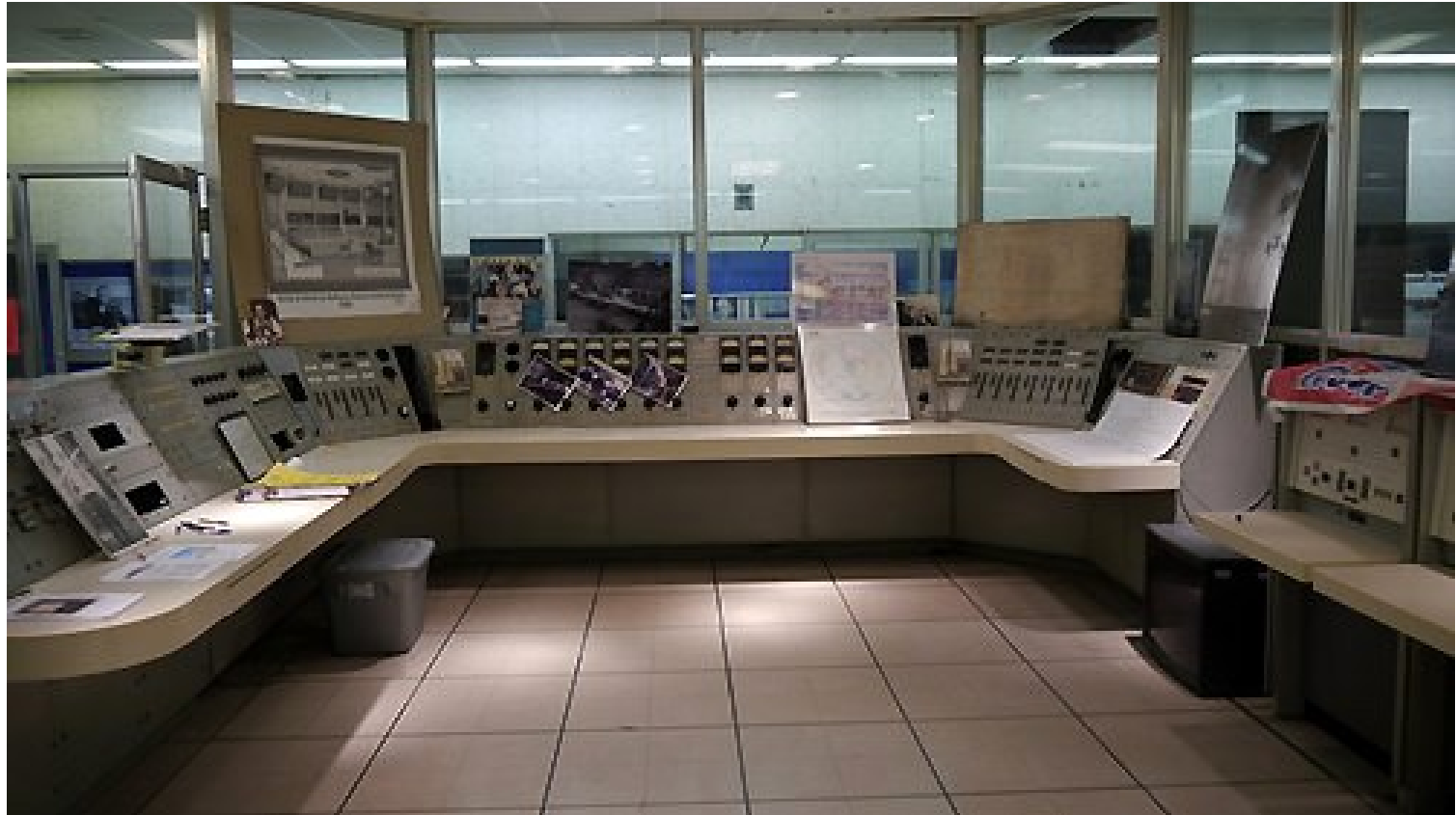
Collins transmitter consoles on right
