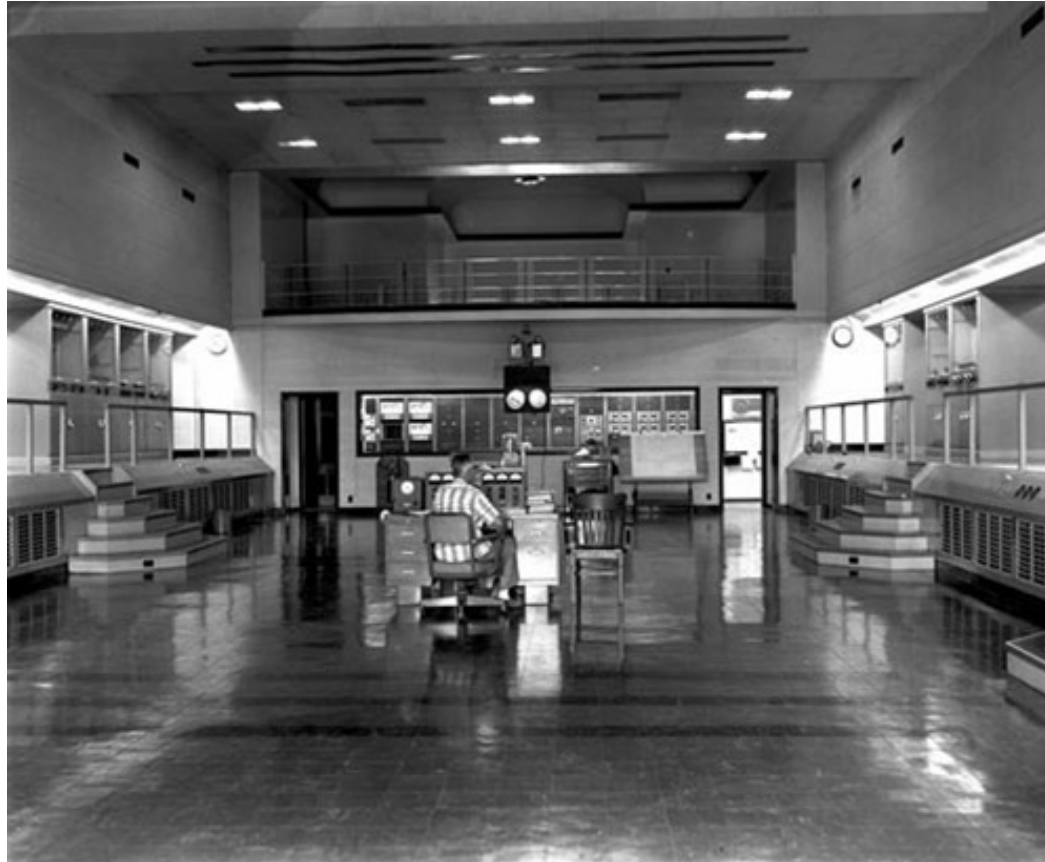
Crosley transmitter bays to left & right of control position
